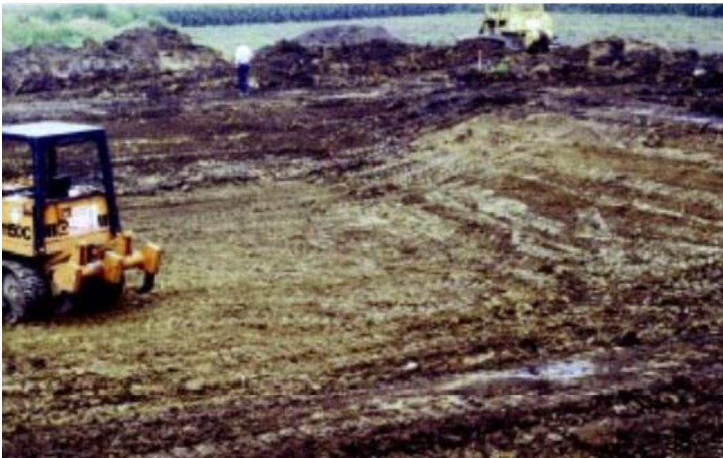
Fig22. The sod and topsoil in a pond construction area can be stockpiled for later use
